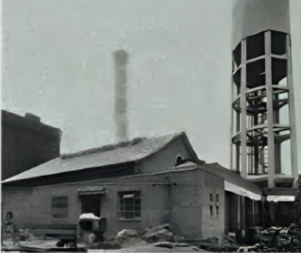
Fig 1. The boiler room under construction in 1940.
